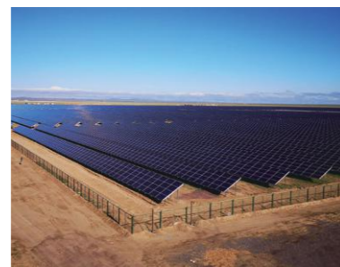
Agadyr Power Plant Kazakhstan System Capacity: 50 MW
