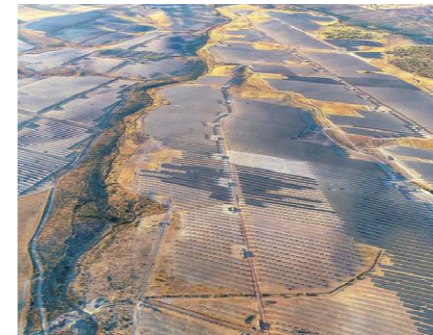
Nuñez de Balboa Power Plant Spain System Capacity: 500 MW (Suntech Supplied 100 MW)
