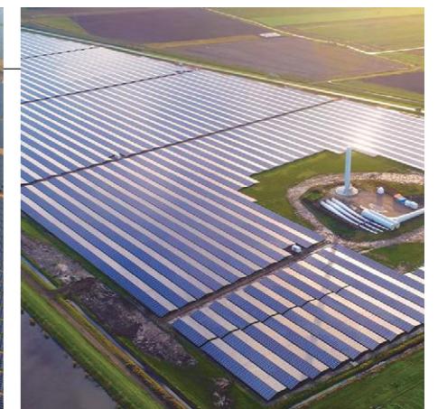
Solarpark Duurkenakker Netherlands System Capacity: 64 MW
