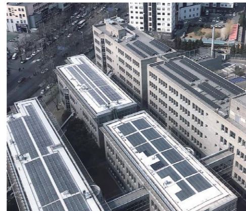
SIEMENS Asia-Pacific Headquarter's Rooftop Project China System Capacity: 308 KW
