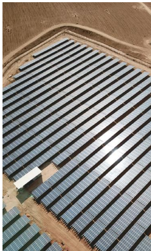
Enlight Kramim Power Plant Israel System Capacity : 18 MW
