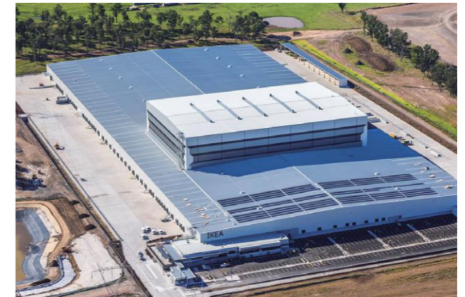
IKEA Rooftop Project Australia System Capacity: 384 KW
