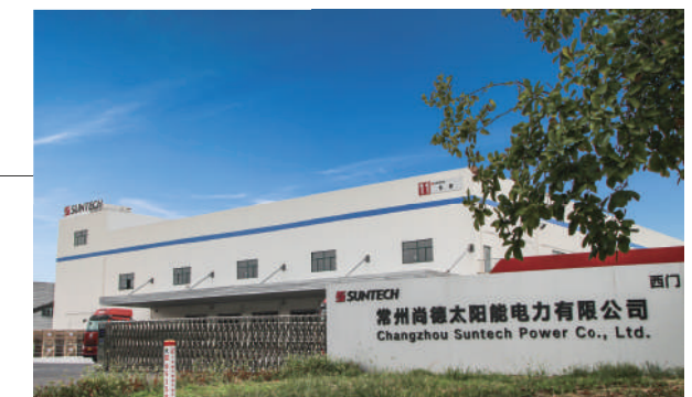
Suntech Power Changzhou Base
